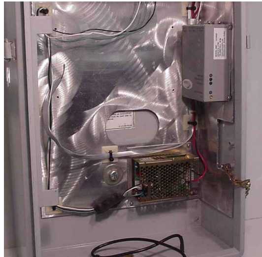
Figure 5 - Plate Installed in Enclosure
