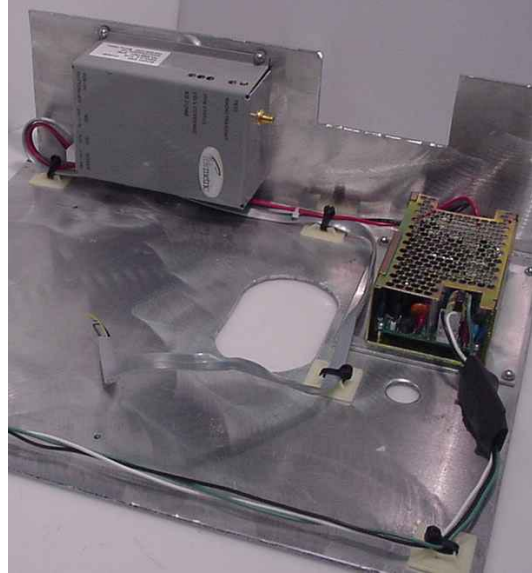
Figure 4 - Wiring Harness Installation
